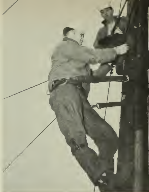
POLE VOLTING—CEs work on line.
